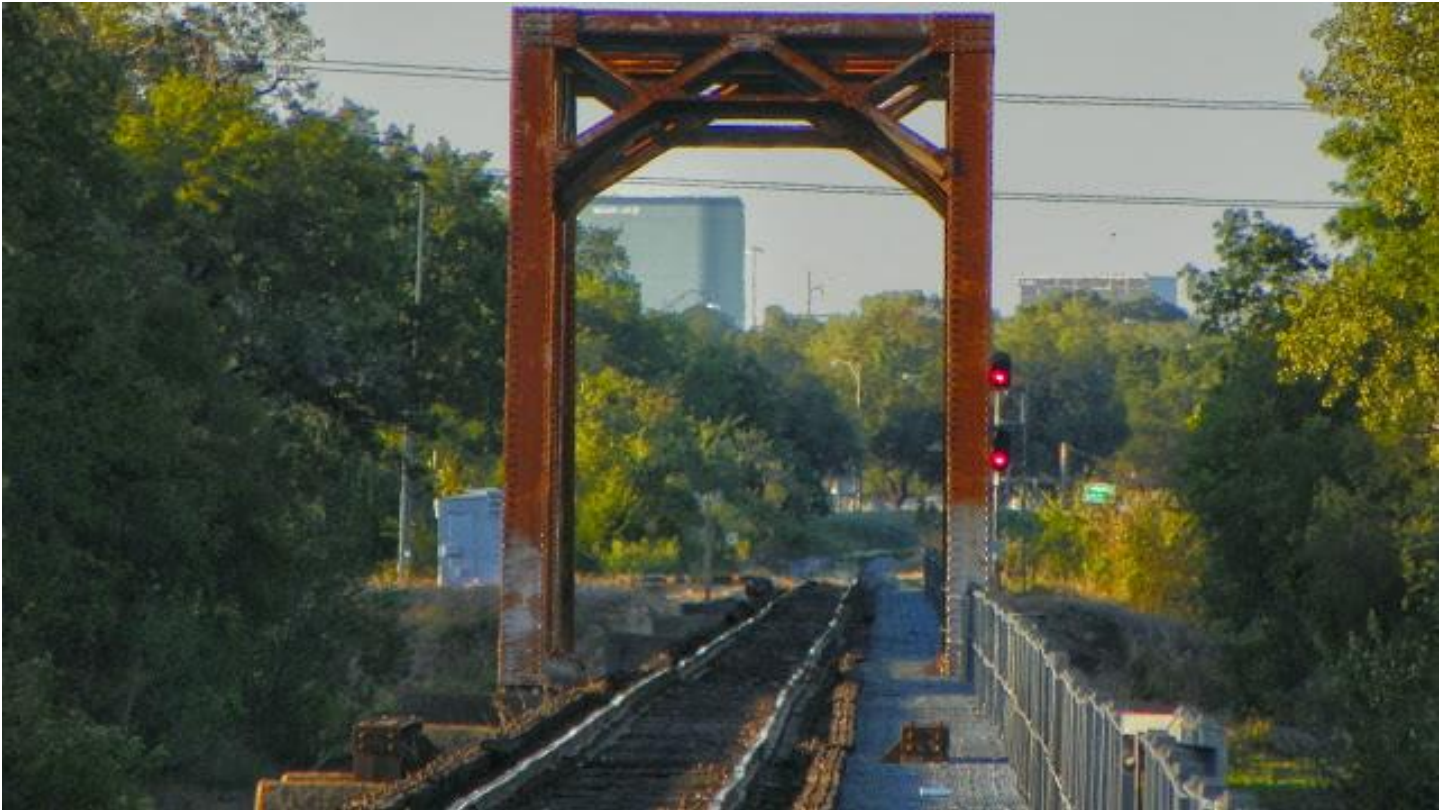
Current Trinity railroad bridge as viewed from Joppa, George Bush Presidential Library and SMU seen in distance
